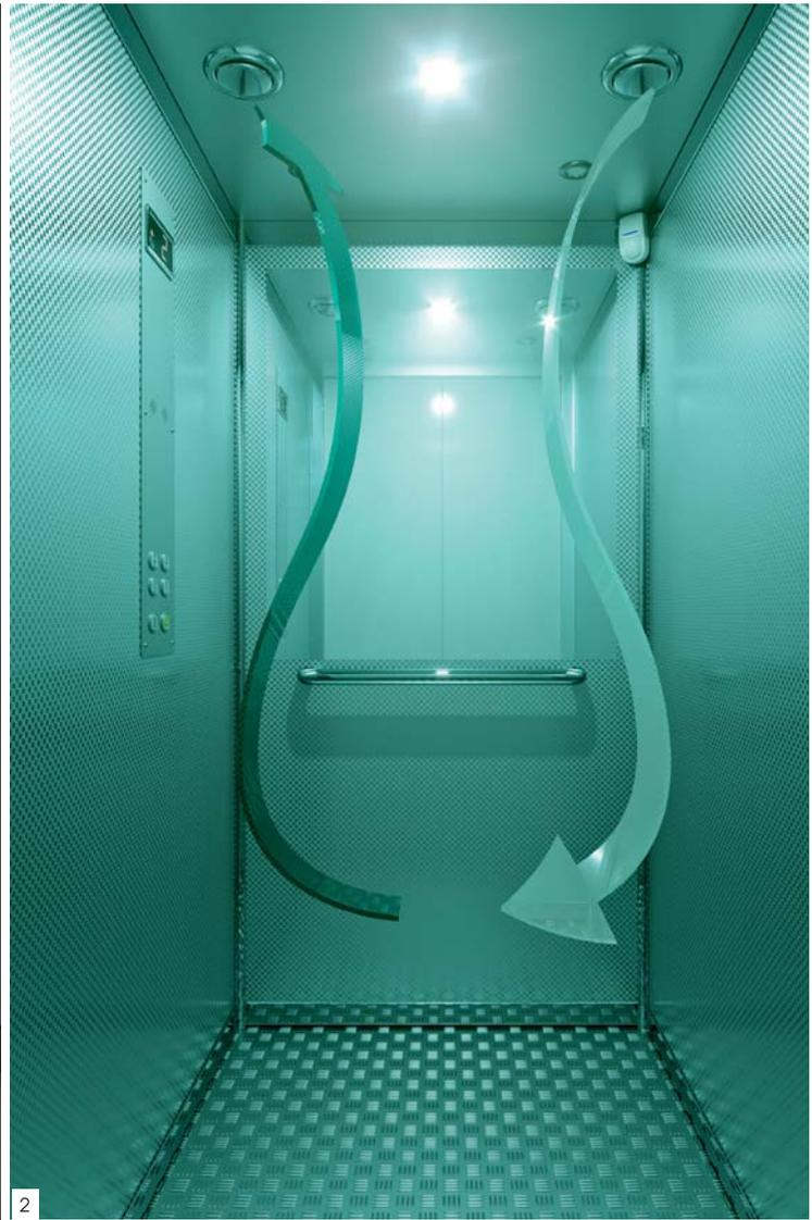
1. Sky Lift, designed by MaMa Design: a virtual opening in the ceiling mimics the visual sensation of the sky and the sun, and the lighting changes with the passing of the day 2. CARE: ventilation scheme with the HEPA absolute air filter
