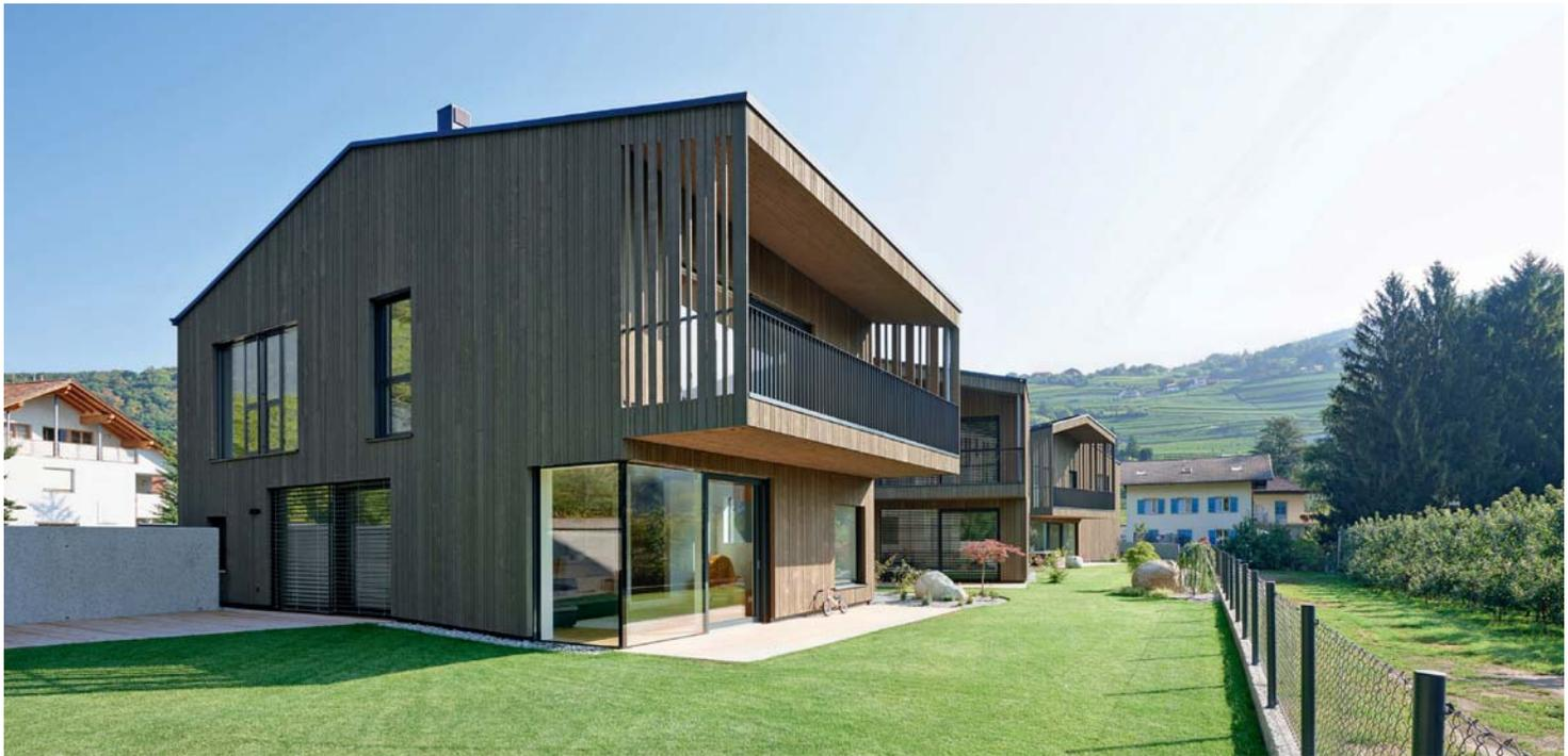
also clad externally with a ventilated façade created using wooden slats.
